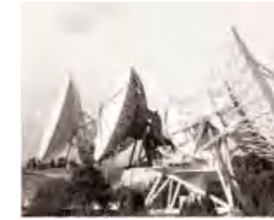
通信设备 Communication Equipment
